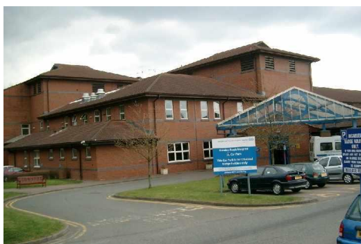
Rowley Regis Hospital, Moor Lane, Rowley Regis B65 8DA
